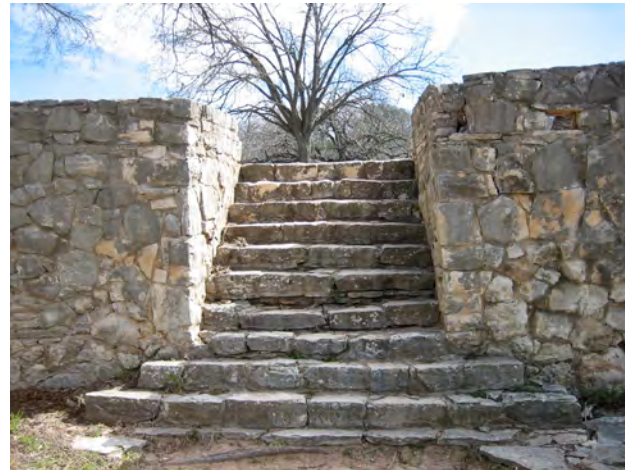
Stone stairs are in disrepair (above and right). Steps should be rehabilitated to improve footing, handrails should be added.
