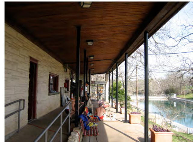
The relocation of the Lifeguard's Lounge/Manager's Office in the 1960s required this elevated passage to account for a level change, changing what was designed to be a shaded social space into more of a passageway.
