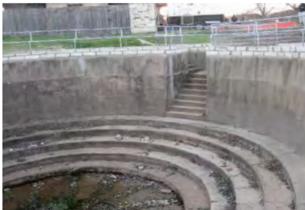
Andrew Zilker's amphitheater has been altered over the years. Note the added band of concrete (the lighter color) and two courses of limestone. This plan recommends returning Eliza to Zilker's 1903 form.
