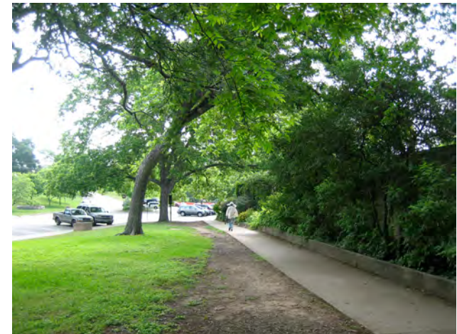
Front Yard grass worn by heavy foot traffic.
