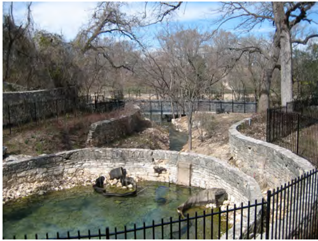
Sunken Garden in 2007. Some walls have collapsed, and the landscape is less organized. The fence is to protect the salamander habitat.
