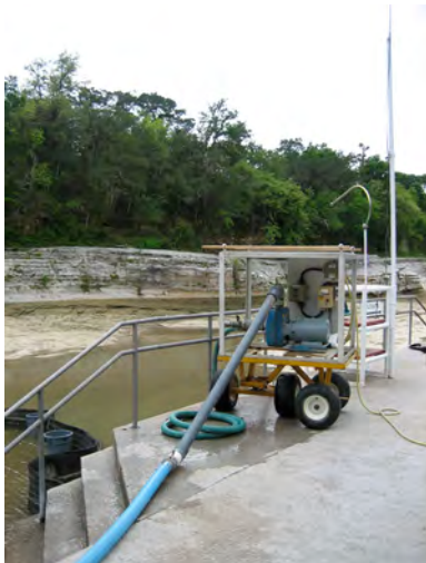
Trash pump used for silt disposal.
