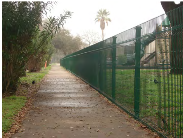
Decorative wire mesh fencing
